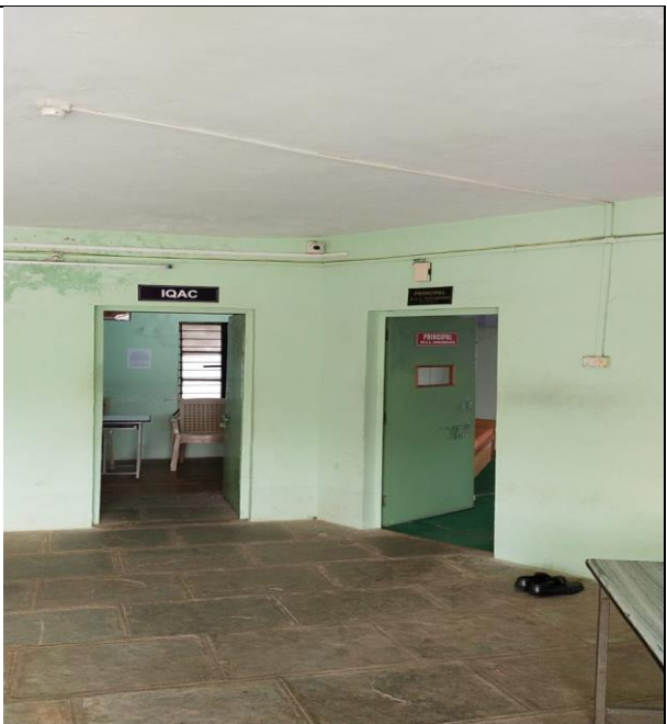
CCTV Surveillane in Principal Cabin
